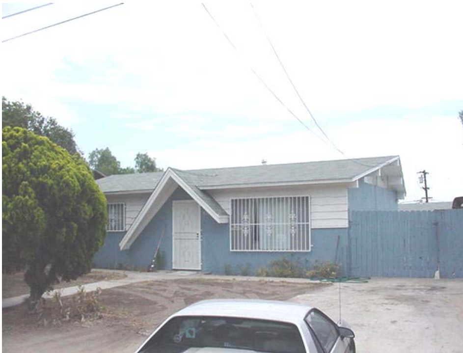
Typical Dwelling Single-Family Residence
